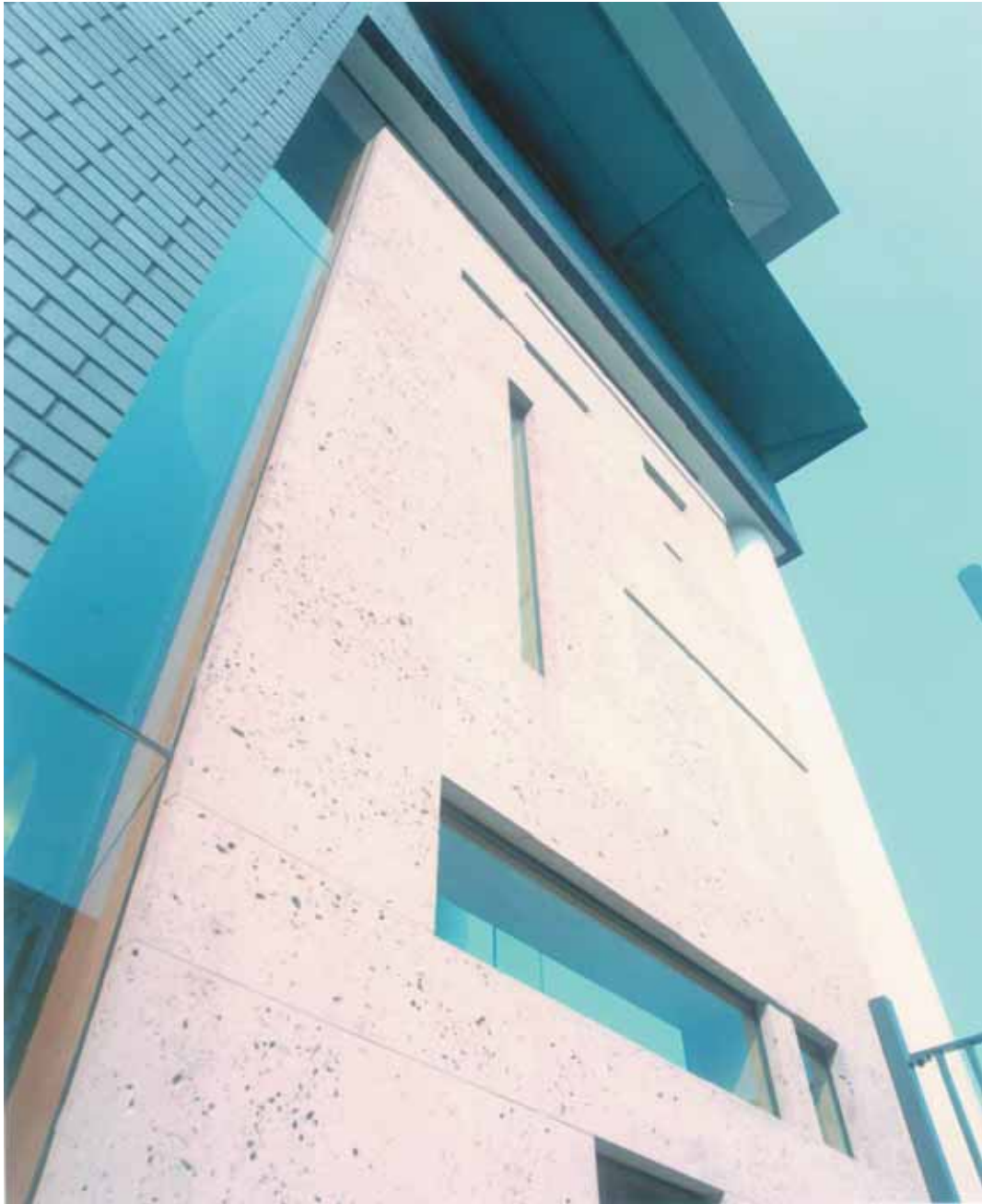
New Bar Library: Robinson, McIlwaine Architects, winner 2004 Civic Trust NI Public Realm Special Award. Photo: Todd Watson
